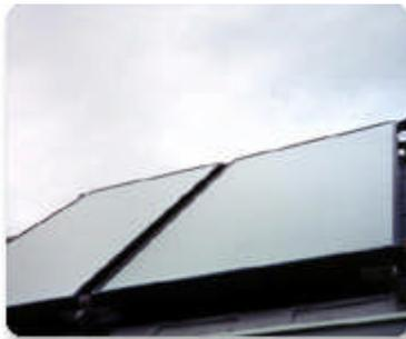
For solar hot water systems, flat-plate solar collectors are typically installed facing south on a rooftop. Credit: James Jones
